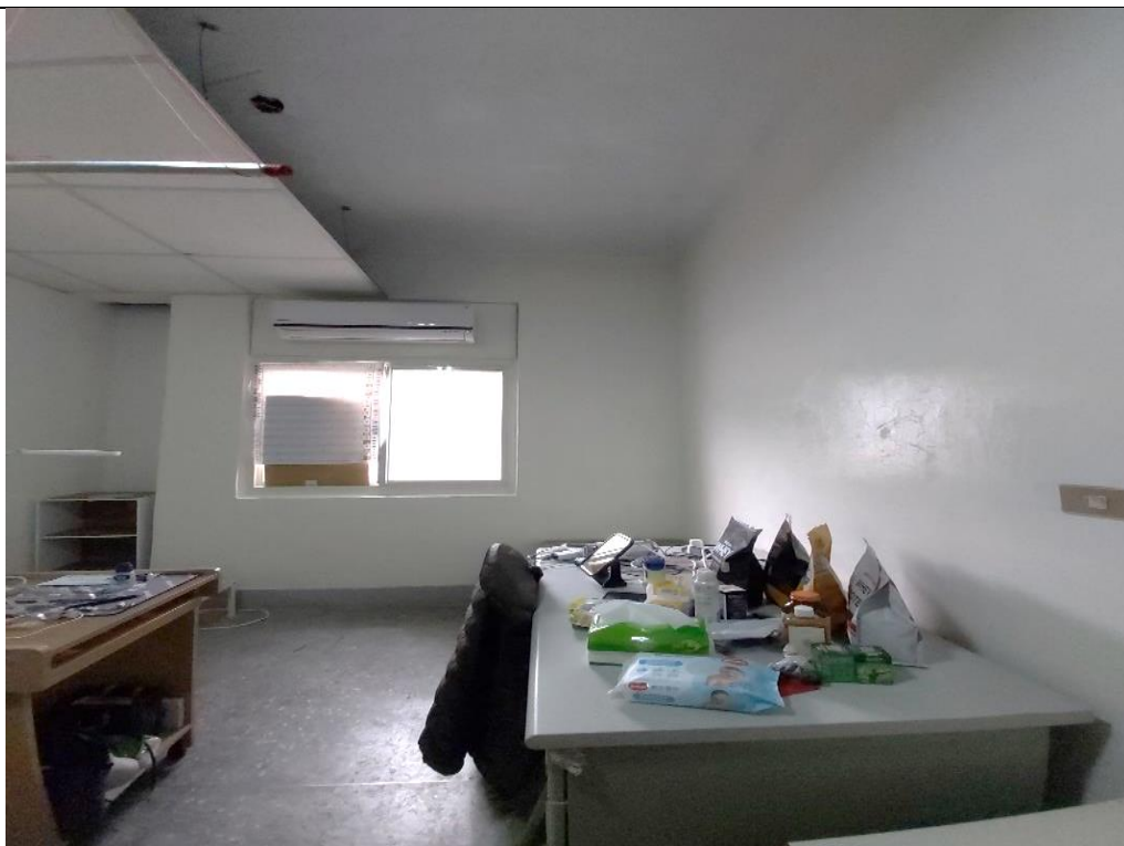
7 (坪林所施工後)
